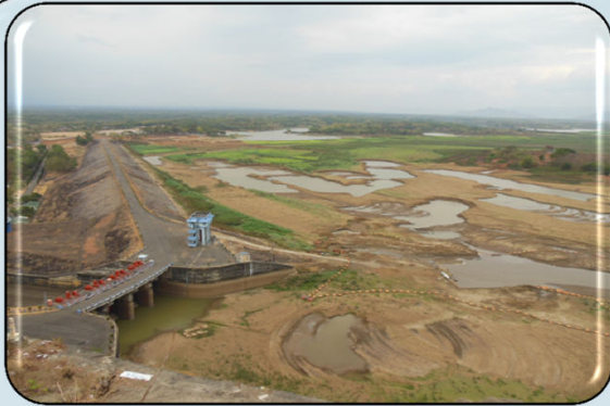
Too Little Water
